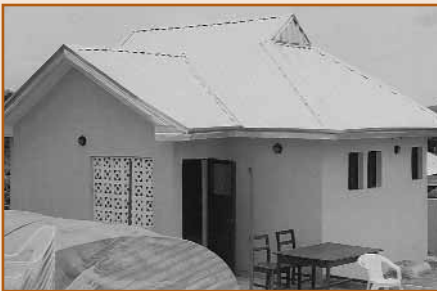
The public library building.
